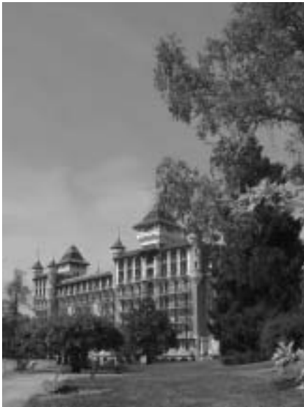
The Caux Conference Centre
